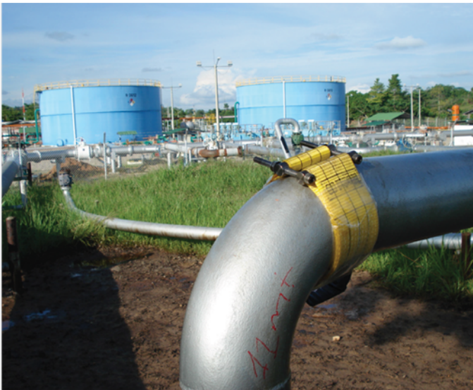
Figure 1. STOPKIT® product installed on an elbow.
