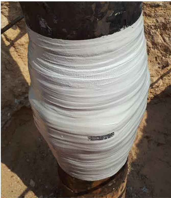
Figure 6. Reinforcement completed and identity plate installed for traceability.
