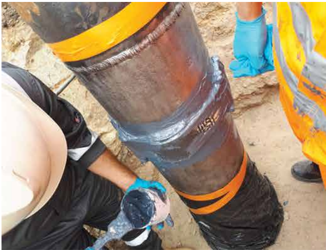
Figure 5. STOPKIT recovered with 3X filler before wrapping with R4D-HT+.
