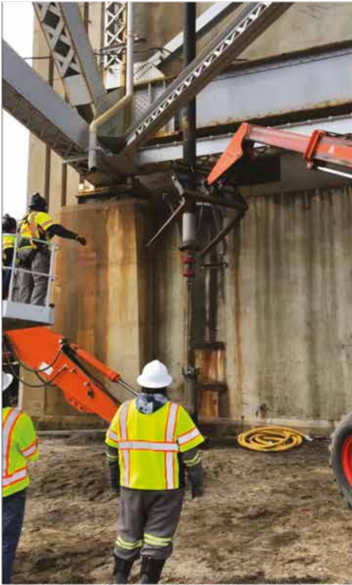
ILI tool being removed from the pipe
