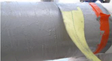
Wrapping in progress ●
