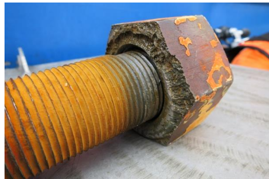
Fig. 4. Damage to studs and nuts (2" diameter)
