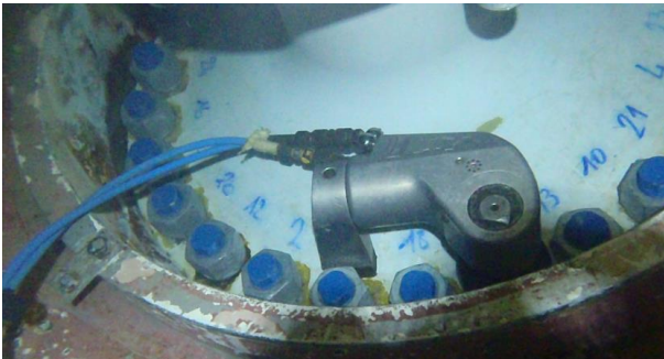
Fig. 30. Torquing tool in position inside the receptacle
