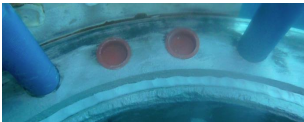
Fig. 27. Application of the composite repair material inside the groove
