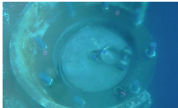
Fig. 28. Mould in place during the curing time
