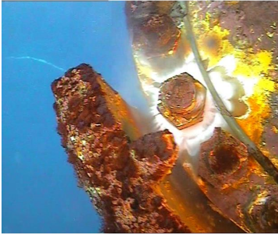
Fig. 1. Leak observed under a nut
