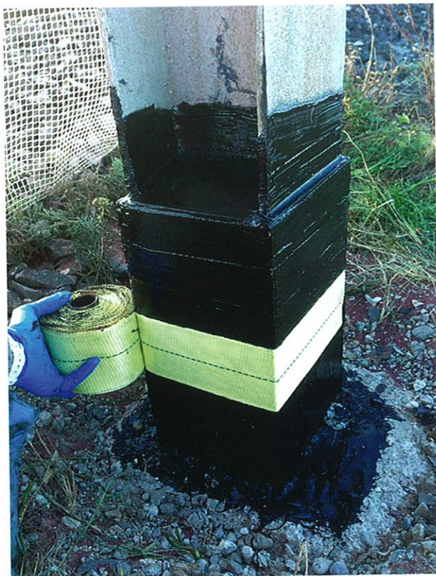
Figure 7g: Wrapping the Kevlar® strip on the repaired mast (step 4).
