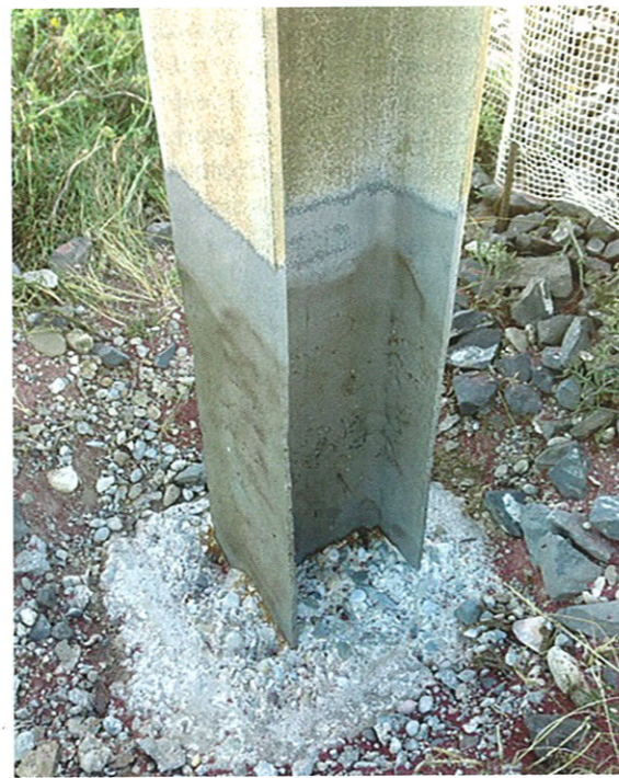
Figure 7b: Mast prepared for repair (step 2).
