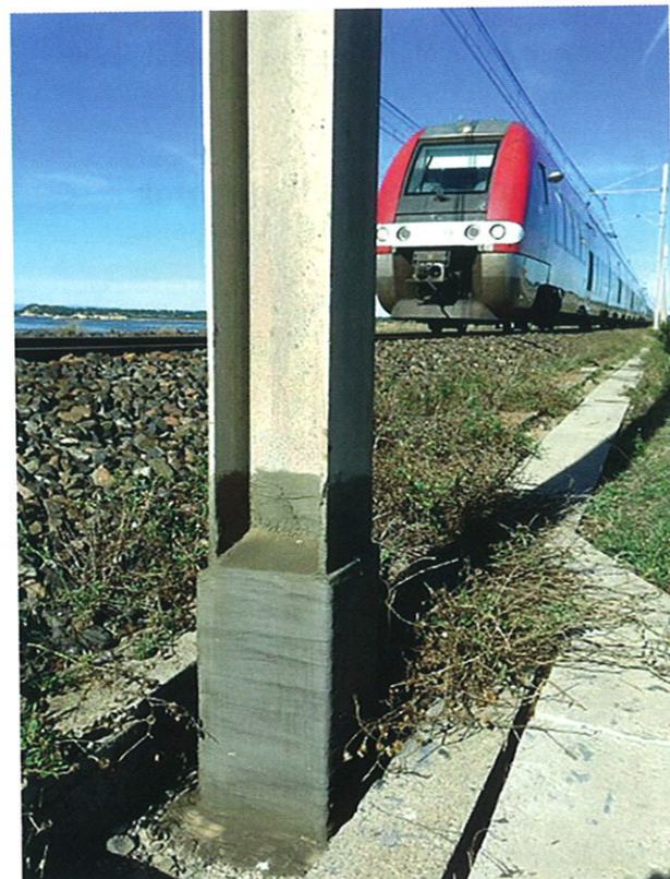
Figure 7h: Repaired mast (step 5).
