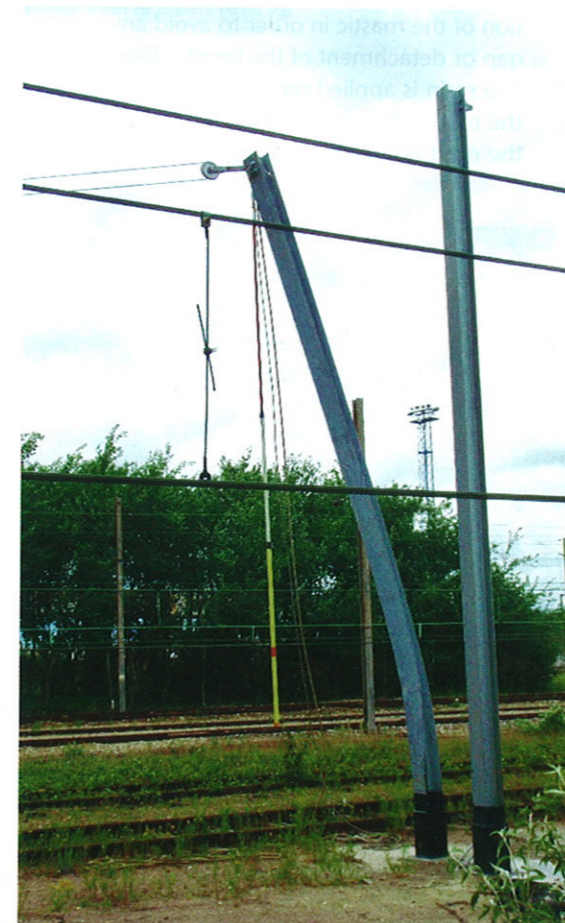
Figure 5a: Testing of a reinforced H-type mast.
