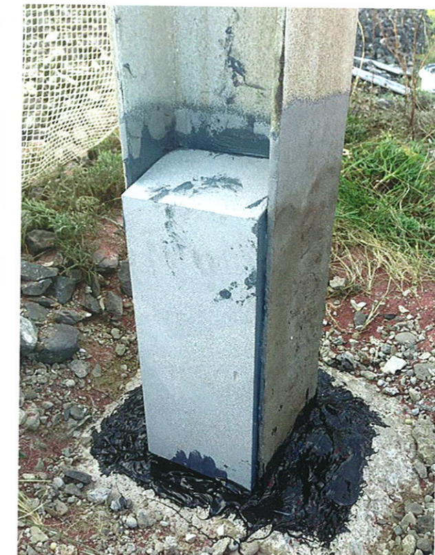
Figure 7d: Reparation of inserts (step 3).
