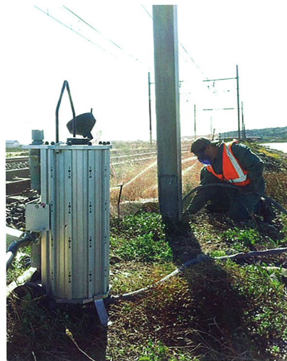
Figure 7a: Preparation of mast surface (step 1).
