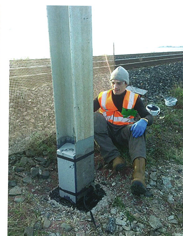
Figure 7f: Application of resin (step 3).
