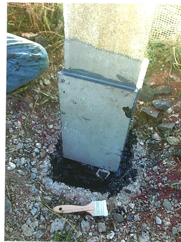
Figure 7e: Polymerization of the mastic (step 3).
