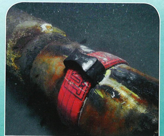
Figure 4. STOPKIT Offshore (online leak sealing).
